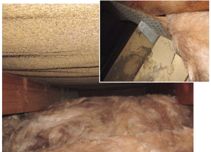
Picture 10 showing the old fashioned roofing felt with inset pic showing the lack of insulation at the eaves.
