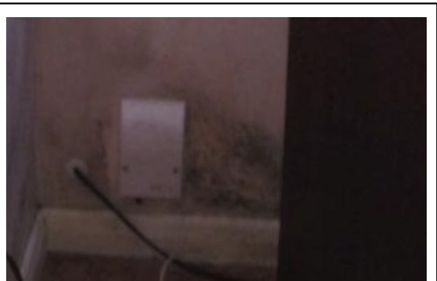
Pictures 7 and 8 show that even socket entry points are cold spots. Corners are particularly vulnerable to mould growth.
