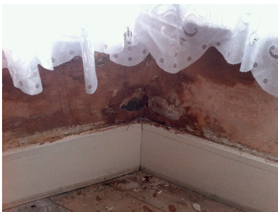
Figure 7: Water penetration through cracked render. Internal wall insulation should not be used to conceal existing issues and should only be applied as part of extensive repairs to the property.
