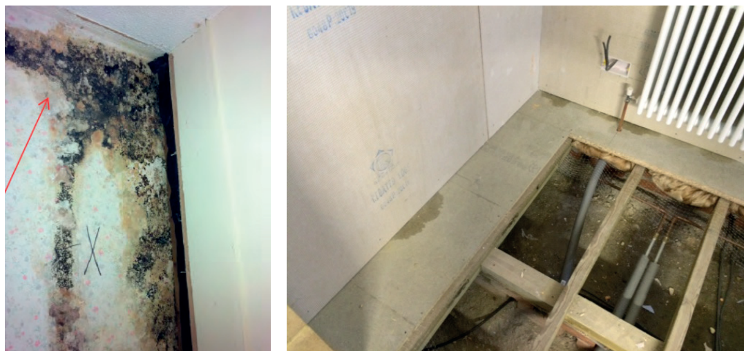
Figure 4: Problems associated with VCL-based insulation systems. (Left) Interstitial mould growth (image courtesy of Simmonds.Mills Architects) revealed during strip out for remedial work. (Right) Condensation accumulation (image courtesy of Acara Concepts).
