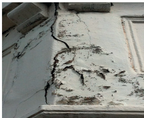
Figure 7: Water penetration through cracked render. Internal wall insulation should not be used to conceal existing issues and should only be applied as part of extensive repairs to the property.
